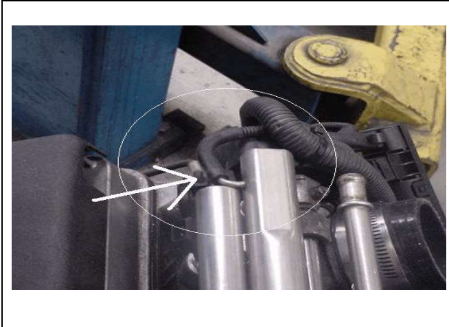
33. MAKE SURE WHERE THE HARD LINE CONNECTS TO THE SOFT RUBBER ELBOW IS TIGHT. IF LOOSE, SECURE IT WITH A LITTLE GLUE OR A TIE STRAP. THIS HARD LINE GOES TO THE FACTORY FUEL PRESSURE REGULATOR AND IT IS IMPORTANT THAT THIS LINE REMAINS CONNECTED!!!
