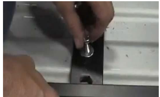
example of plusnut being compressed
